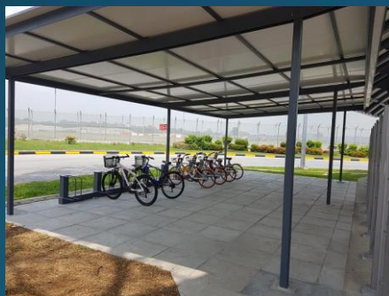
Installed brand-new bicycle parking zone to facilitate cyclist needs.
