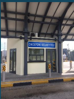
Constructed a brand-new guard-post to facilitate bus security checks.
